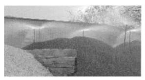
Sprinkling Aggregate in a Stockpile
